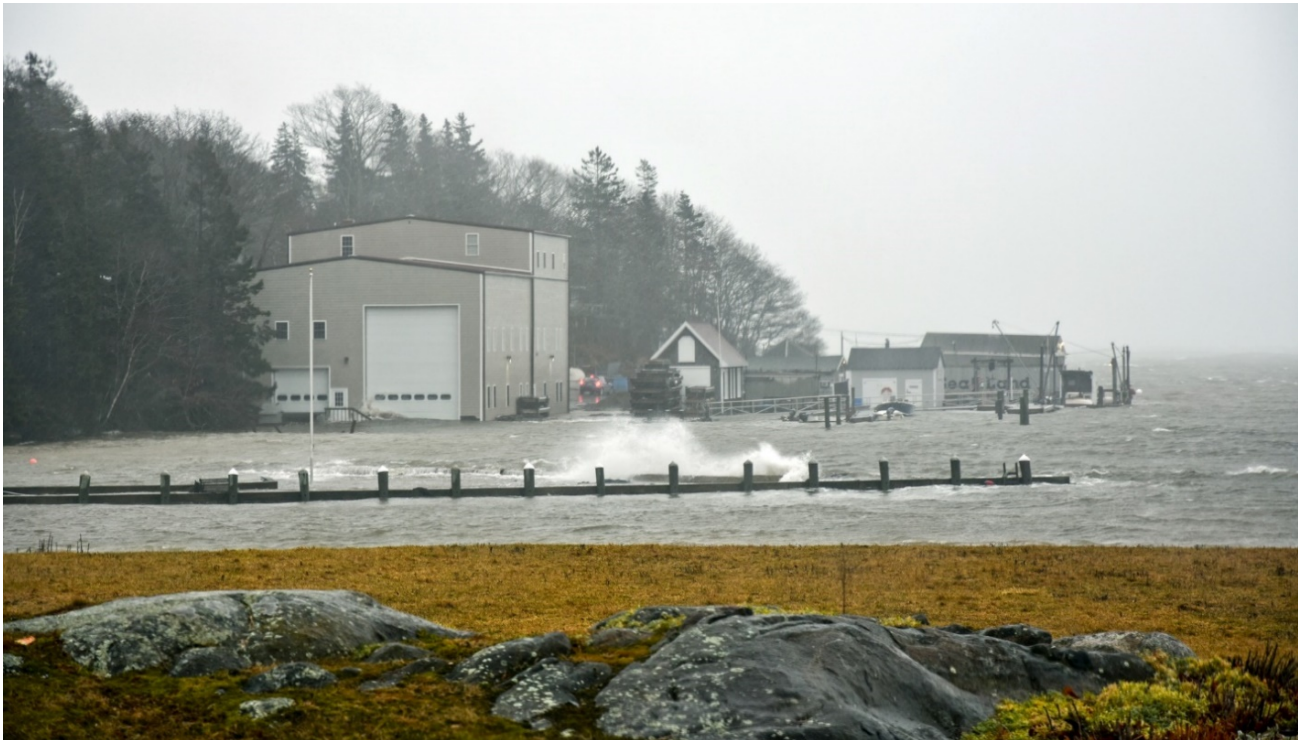
January 2024 storm in Tenants Harbor showing storm surge inundation on commercial wharves Photo: Hal Oaks
